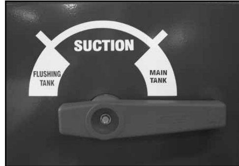
(3) Suction Selector Valve set for the main tank.
