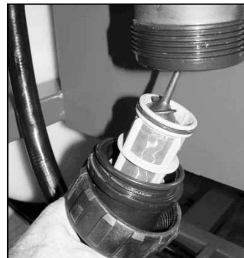
Check the pressure filters are clean.
