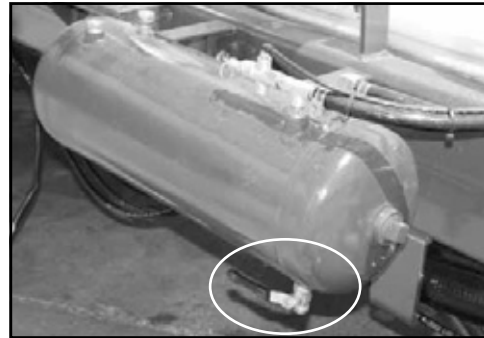
Air chamber drain valve/tap.
