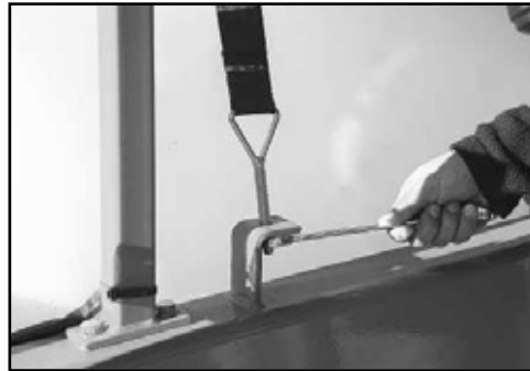
Regularly check that tank straps are tight.
