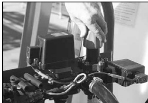
Adjust the manual pressure relief valve.
