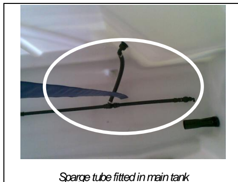
Sparge tube fitted in main tank
