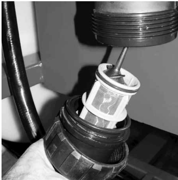
Check the pressure filters are clean.
