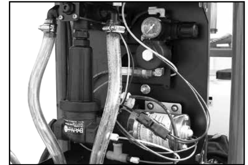
Use an air hose clean out the cabinet area.
