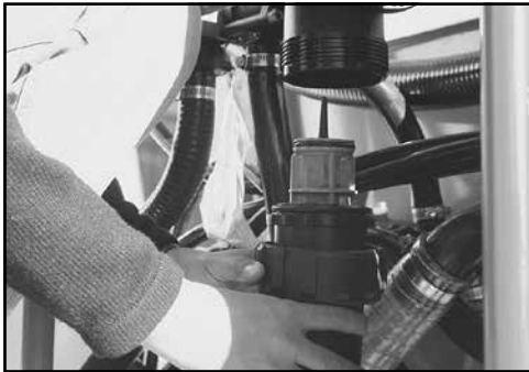
Check the pressure filter is clean.
