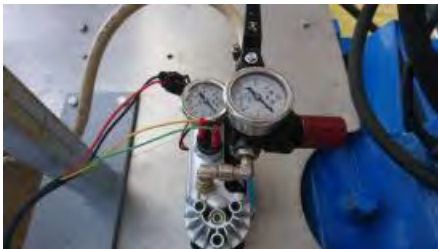
Figure 2-2 Air compressor feeding the PAV valve with compressed air.
