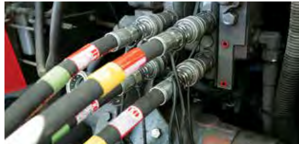
Disconnect hydraulic hoses
