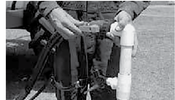
Open Probe valve to transfer mixture to spray tank
