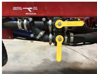
GRANULE INDUCTOR DIVERSION VALVES
