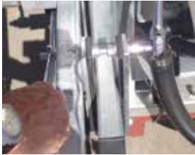
Fig 9: Do up the nuts to hold your new setting in place.
