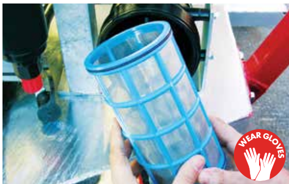
Remove & clean the filter element & components
