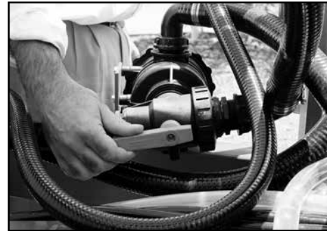
(b) Turn directional valve to source from spray tank.
