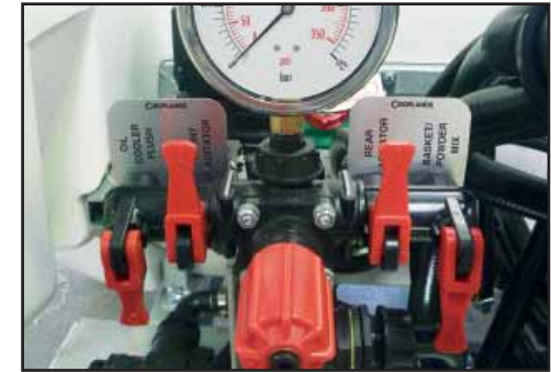
Agitator valves OPEN & mixing basket valve CLOSED.
