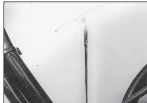
Rear clamps of the main tank.
