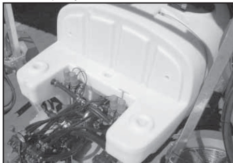
Completely remove the fresh water tanks.
