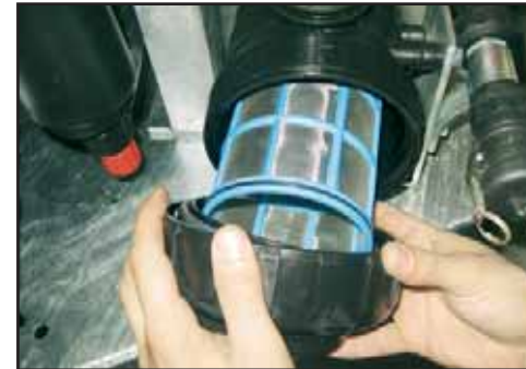
Remove & clean suction filter screen and reassemble.
