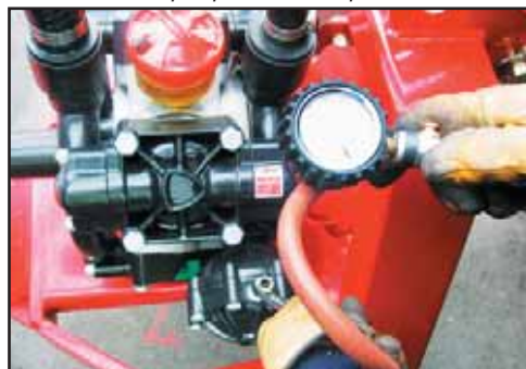
Check pump air chamber pressure.
