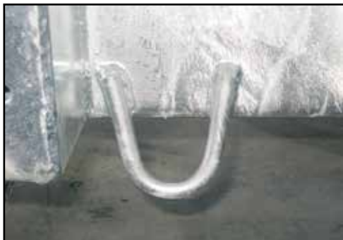
Use tie-down points provided when transporting.
